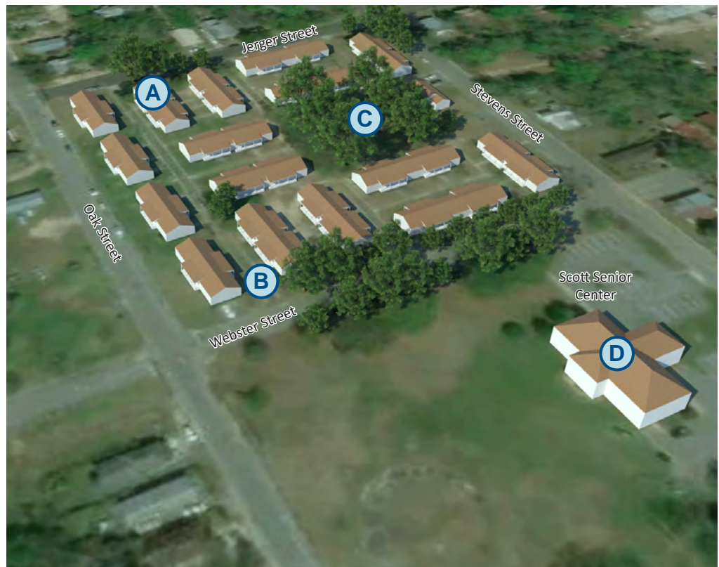
Faircloth Homes: Existing Conditions Aerial
