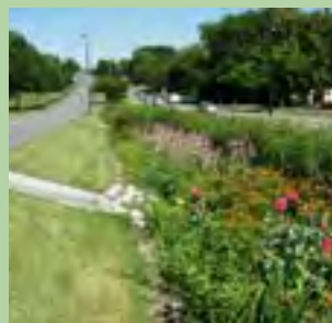
T2-T3: Bioretention swale
