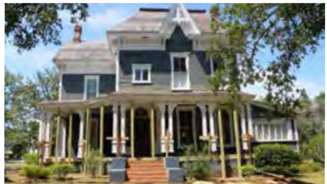
Historic Home Undergoing Restoration
