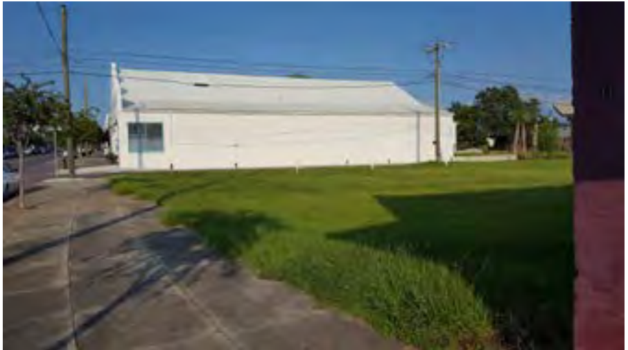
Temporary Interventions: Existing Conditions
