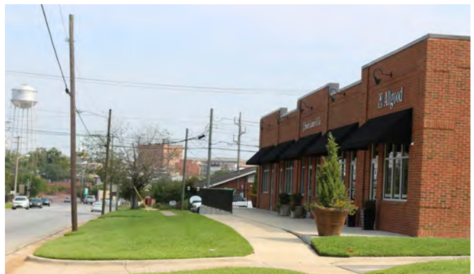
New Commercial on Jackson Street
