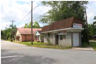
Vacant commercial building
