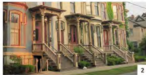
Figure 3-8: Examples of stoops 1. Unroofed stoops 2. Covered Stoops
