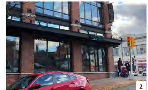
Figure 3-5: Examples of shopfronts and details 1. Shopfront with a recessed doorway 2. Shopfront with metal Canopy
