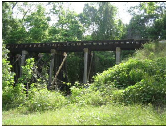
Existing Railroad Trestle
